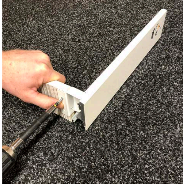
Fit the drawer rear using 16mm screws
