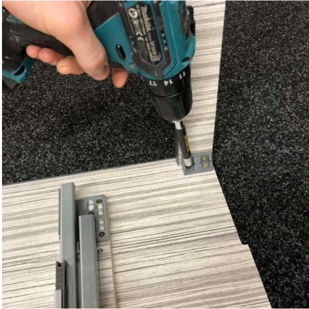
Fit the drawer upper support to the fridge pod (L)
