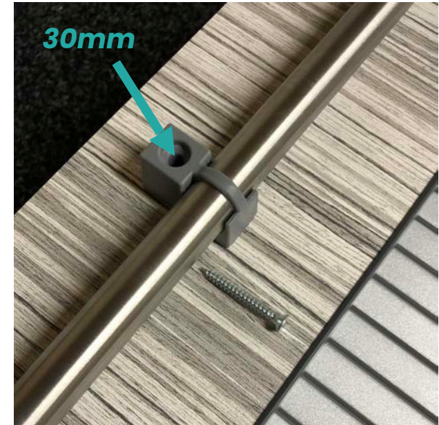
Fit the centre support using a 30mm screw
