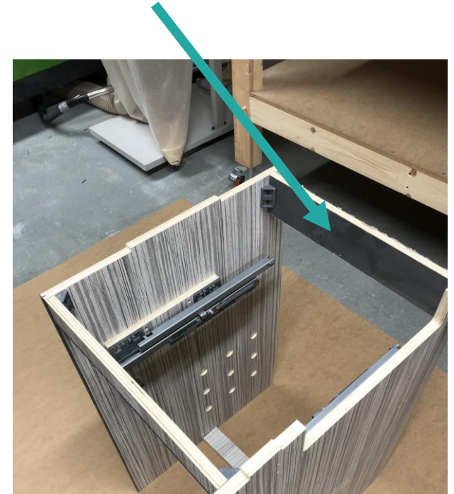
Fit the unit rear support over the finger joint of the fridge pod (R) and chock block to fridge pod upright (L)
