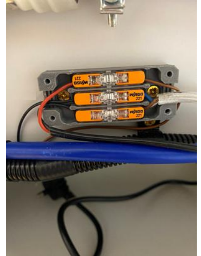
Connect the tap, water pump and top loom wires using 3 x labelled wago connectors- see diagram on next slide
