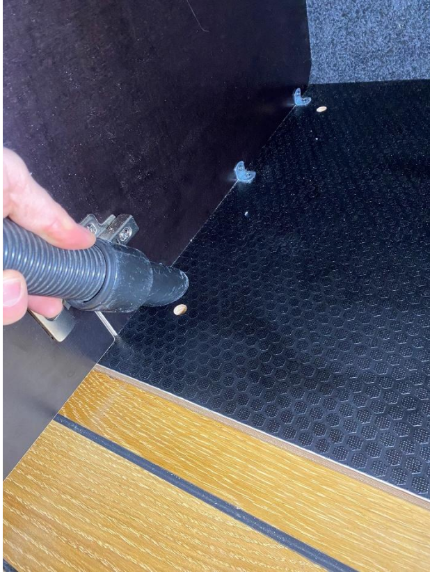
Clean the hole out using a hoover
