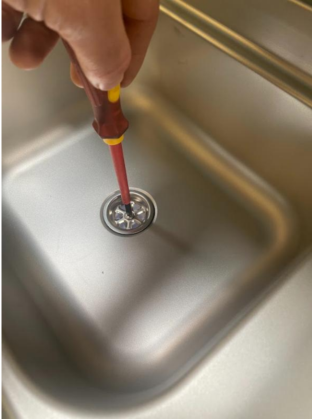
Screw the drain into place
