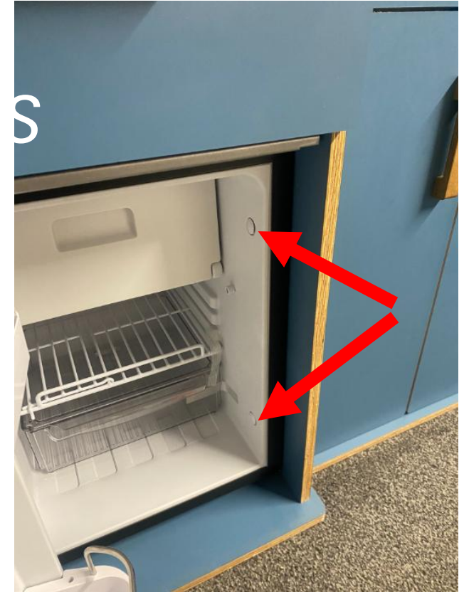
Screw through the right side into the aperture, use 25 or 30mm screws, be mindful not to screw through the ply
