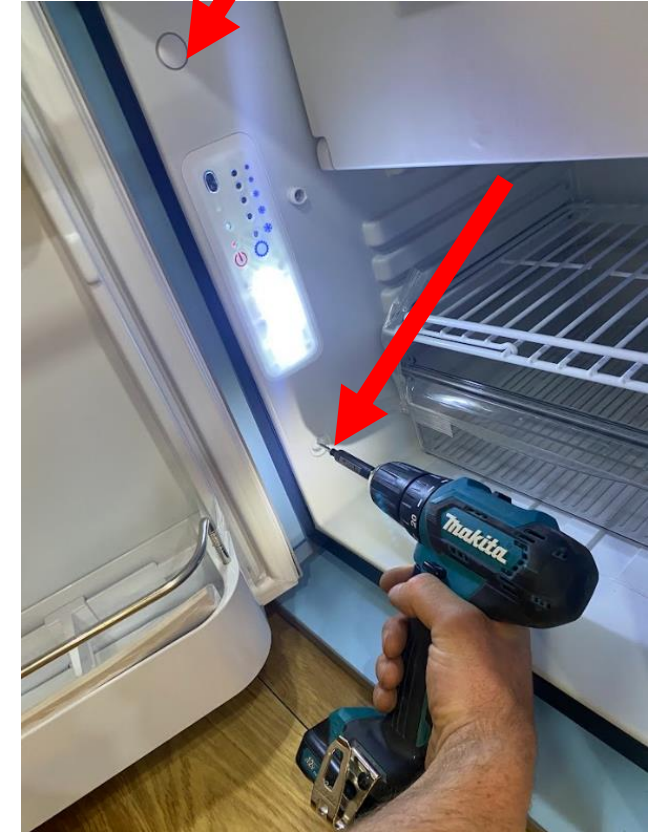
Remove the fridge fixing point caps, screw though into the aperture, use 25 or 30mm screws, be mindful not to screw through the ply
