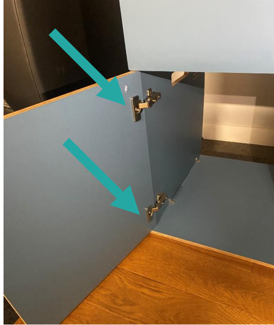
Fit the fridge door using overlay hinges
