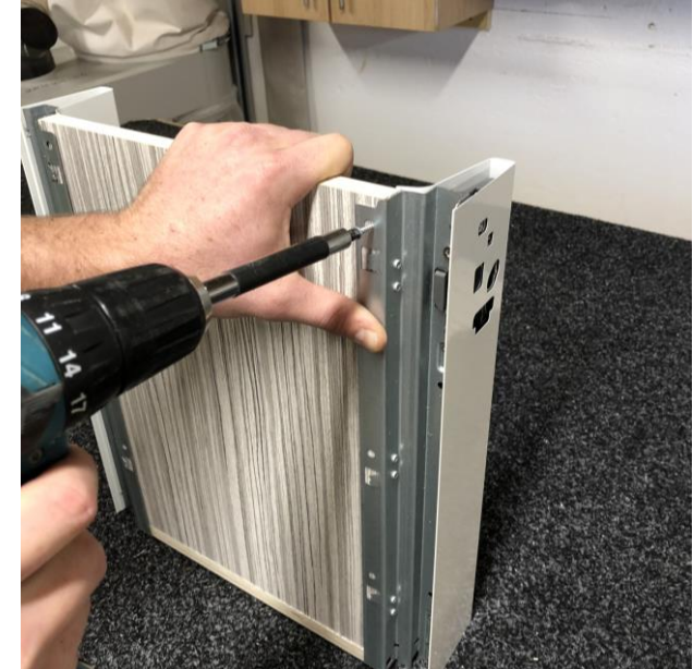
Fit the drawer base using 15 mm screws, ensure the base is flush to avoid gaps
