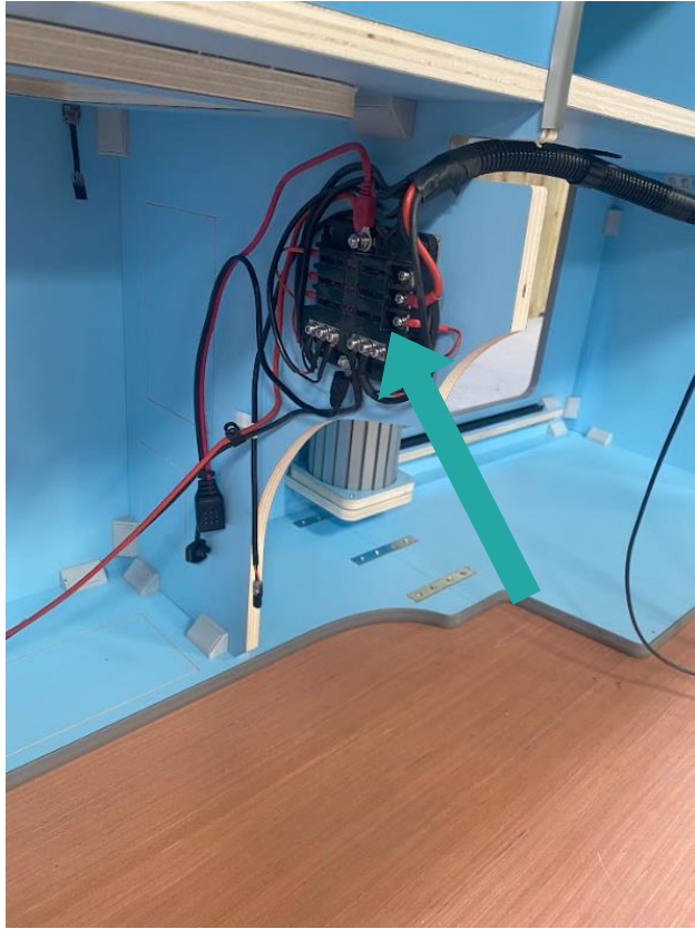
Screw the fuse board into place using the pilot holes provided
