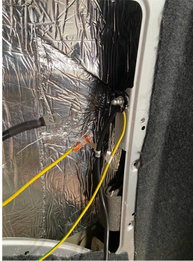
Fit the earth cables
