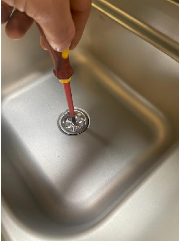
Screw the drain into place
