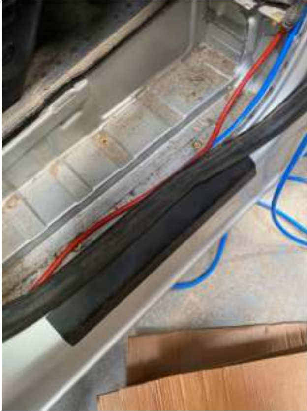
Continue to feed the cables along the sidestep
