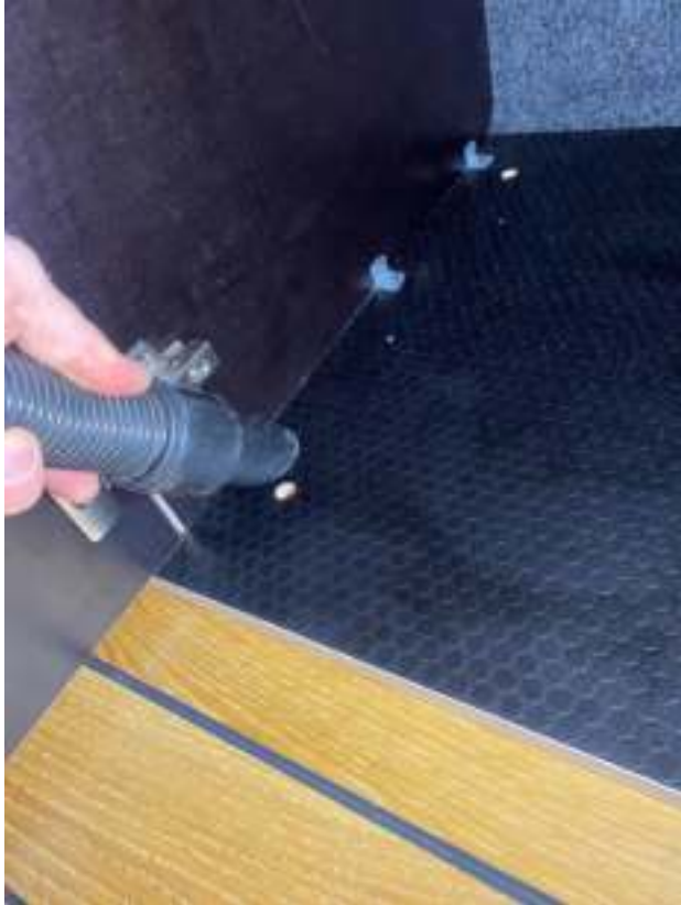
Clean the hole out using a hoover
