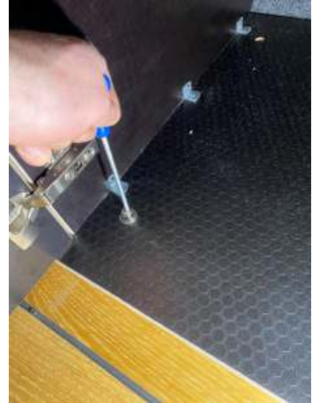
Secure with a 25mm washer and 30mm M6 bolt. Repeat the process
