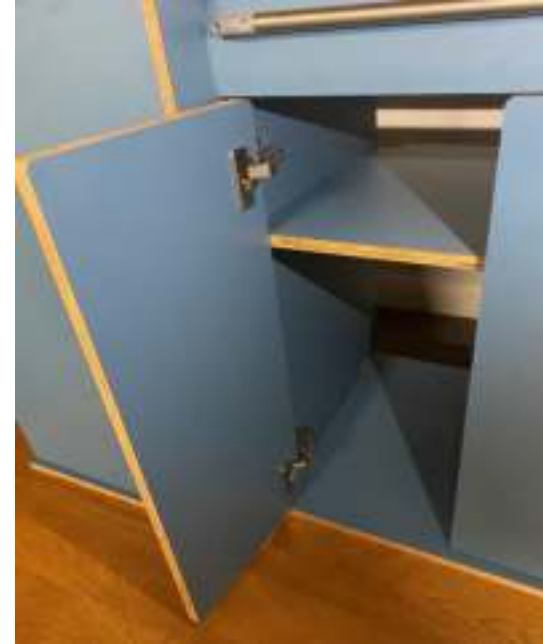
Fit the left under sink door B3 using inset hinges
