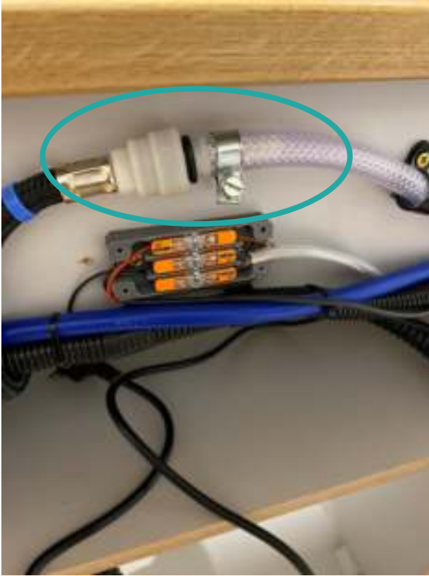
Connect water pipe to tap, secure with jubilee clip
