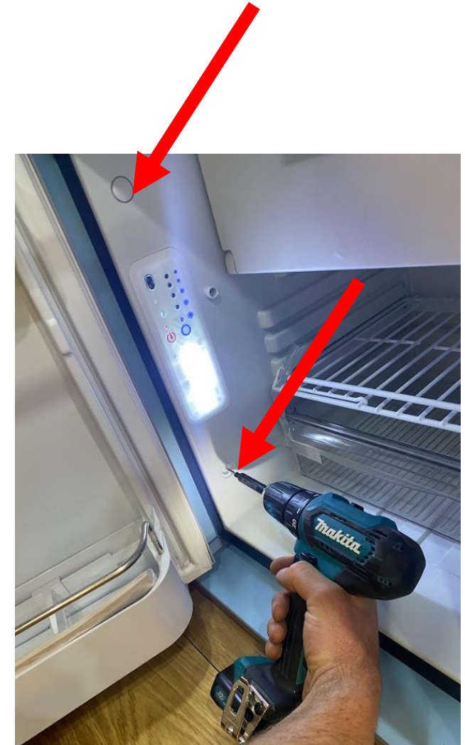
Remove the fridge fixing point caps, screw through into the aperture, use 30mm screws, be mindful not to screw through the ply
