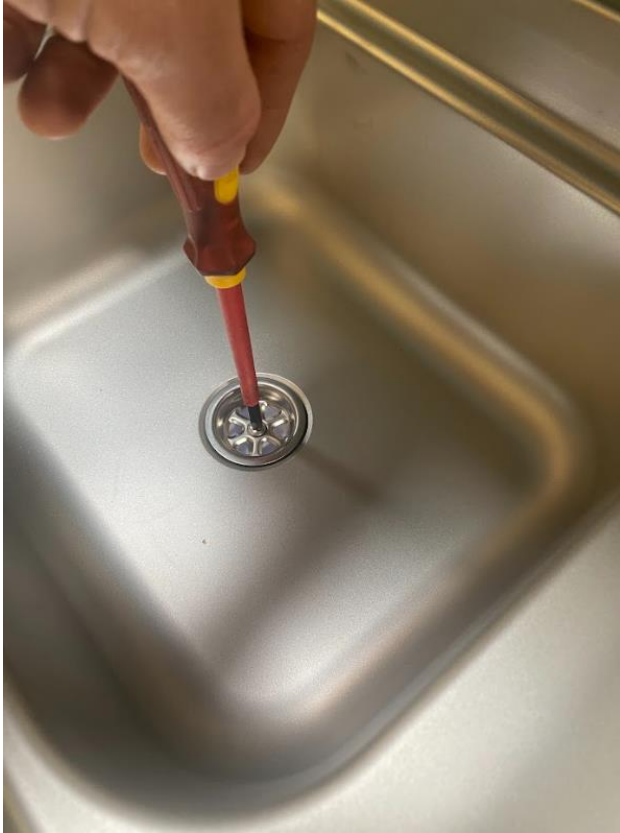
Screw the drain into place
