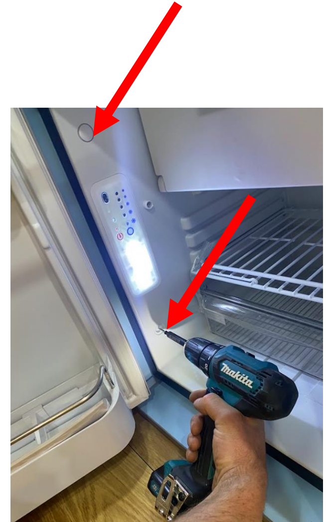
Remove the fridge fixing point caps, screw though into the aperture, use 30mm screws, be mindful not to screw through the ply
