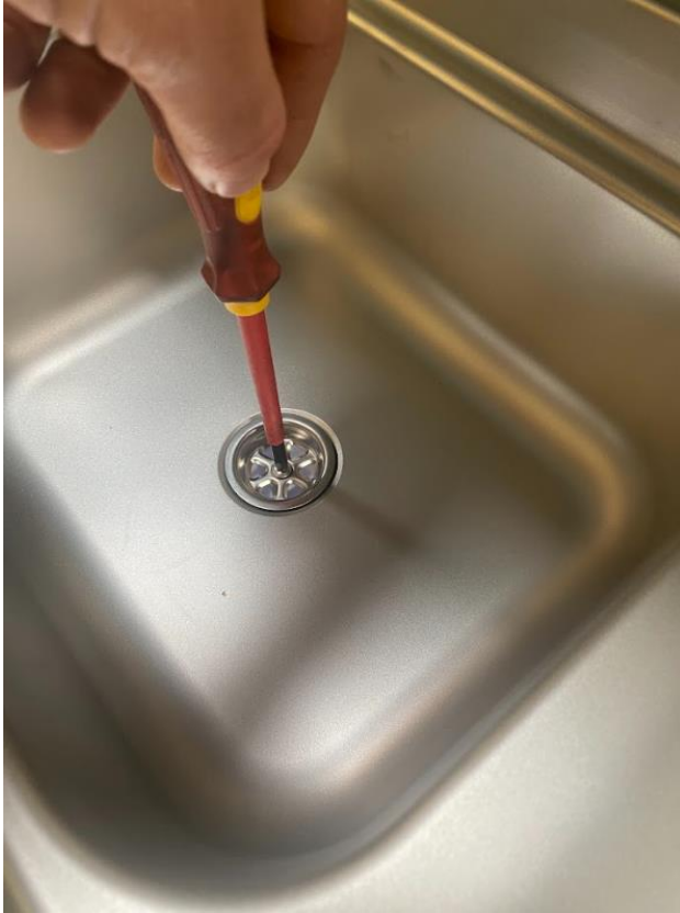
Screw the drain into place
