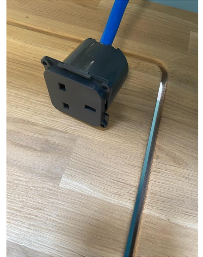
Re attach the back cover of the 240 C-line socket
