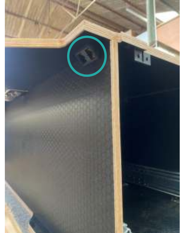
Continue to the rear, ensure to use this block for width alignment
