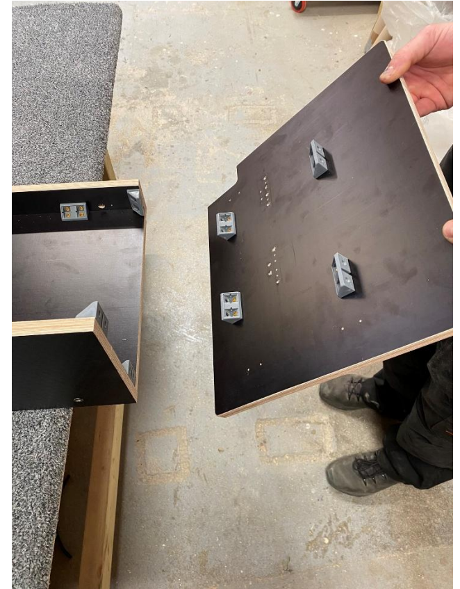
Fit A10 as per picture using pilot holes to align
