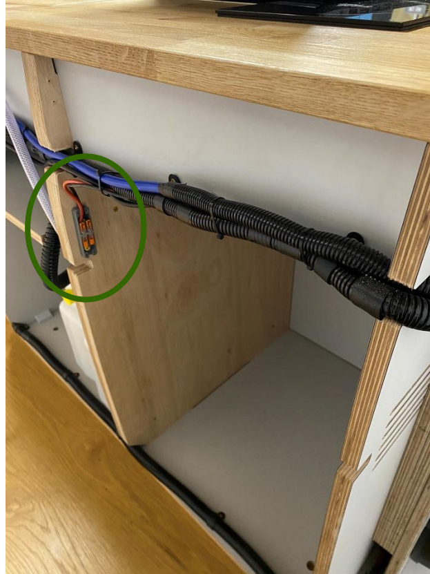
Insert fridge cables from the top loom into a 2-way wago junction box and screw into position as per picture
