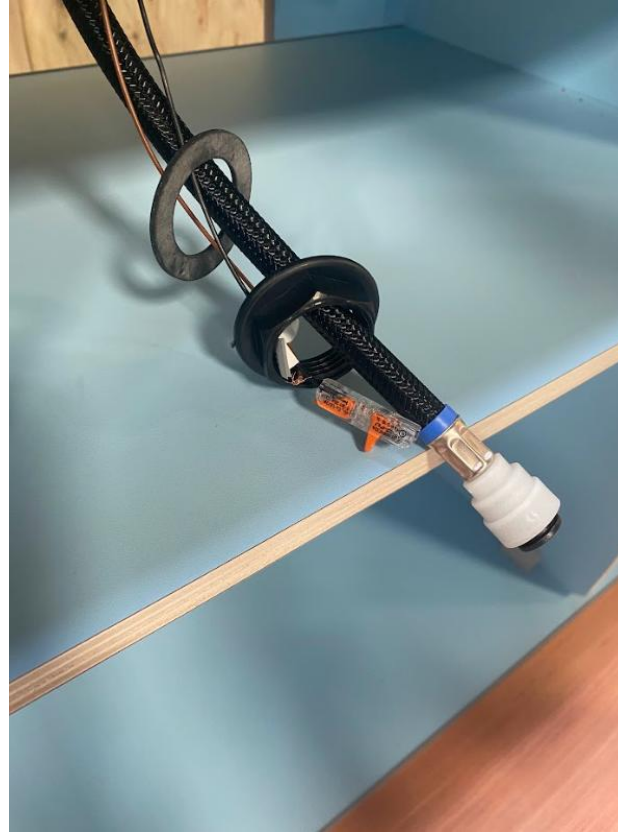
Feed the rubber seal then fixing thread over the water pipe and cables from behind and tighten
