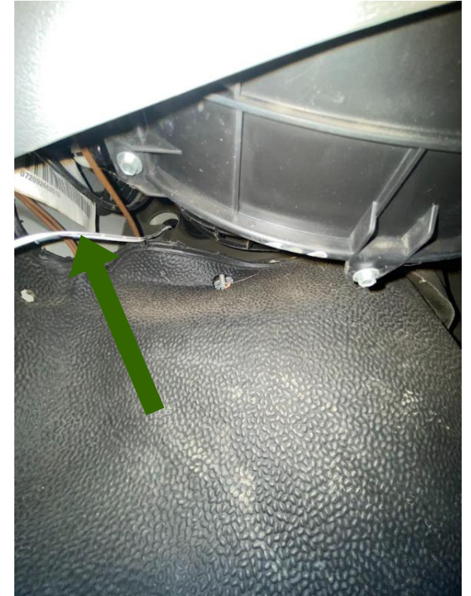
Feed some guide wire through the hole to establish the path, we have used some old BT cable in the picture
