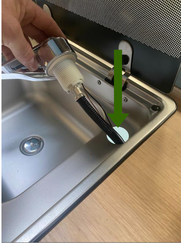
Feed the tap through the tap hole
