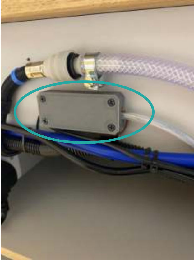
Fit the 3-way wago junction box and cover
