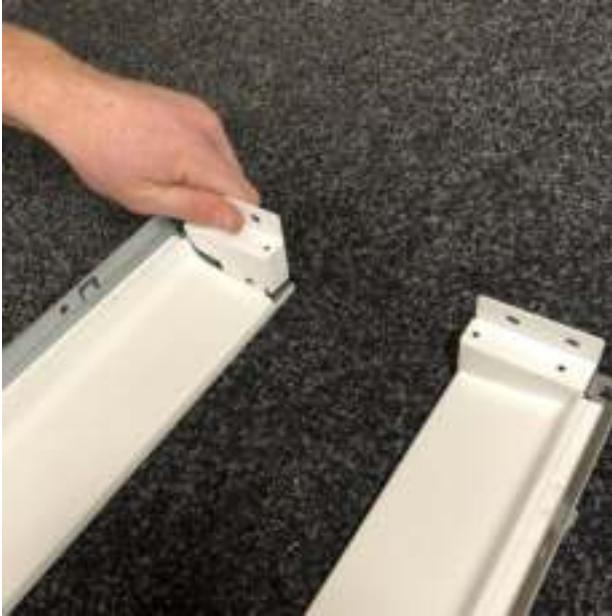
Attach the mounting clips
