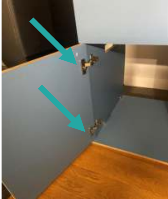
Fit the fridge door A3 using overlay hinges
