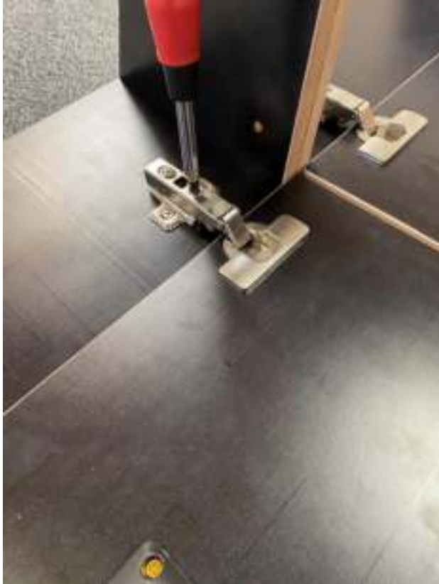
Adjust the hinges to suit
