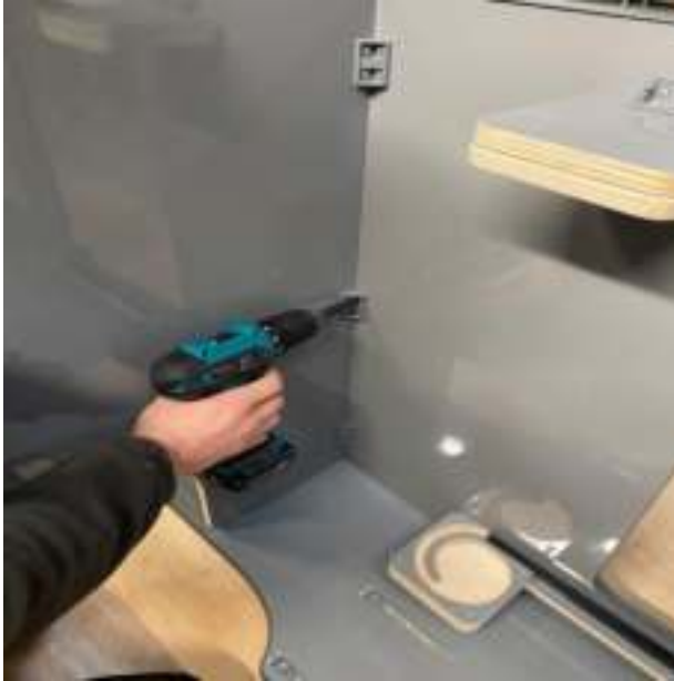
Fit the Kitchen unit face B1 from the rear
