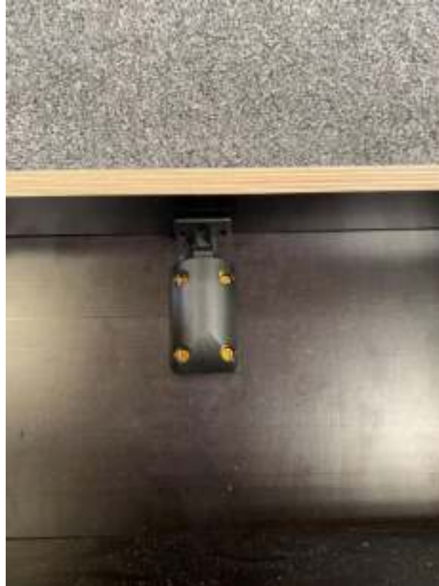
Fit strike plates for the handles
