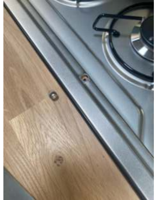
Insert the grill to the underside template. Fit the screw inserts
