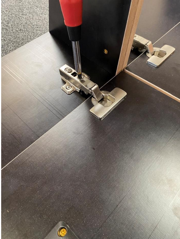
Adjust the hinges to suit
