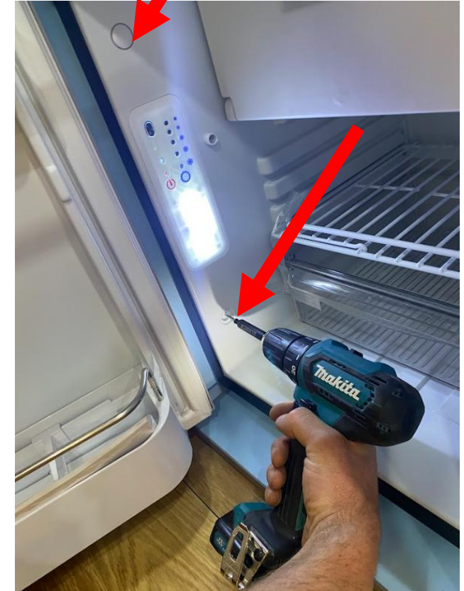
Remove the fridge fixing point caps, screw though into the aperture, use 30mm screws, be mindful not to screw through the ply
