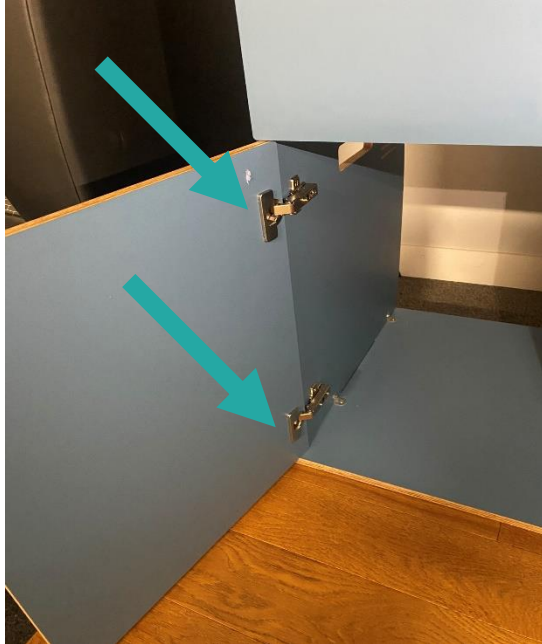
Fit the fridge door using overlay hinges
