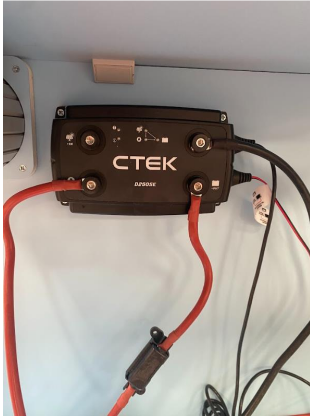
Screw the CTEK split charge into position
