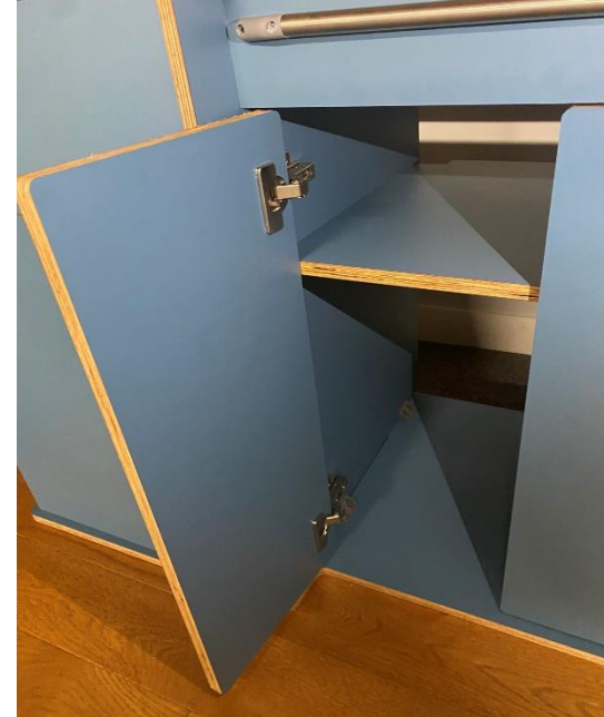
Fit the left under sink door using cranked hinges
