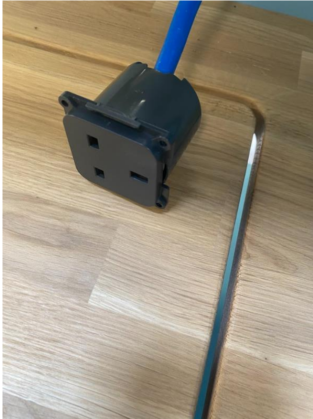
Re attach the back cover of the 240 C-line socket
