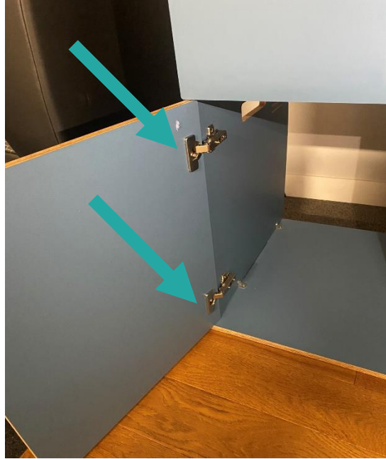
Fit the fridge door using overlay hinges
