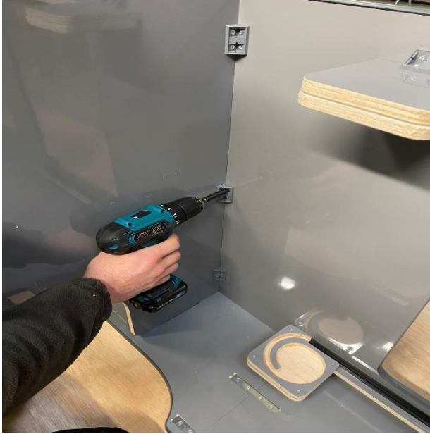
Fit the Kitchen unit face from the rear
