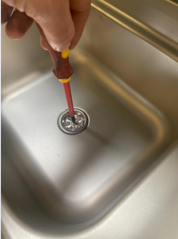
Screw the drain into place
