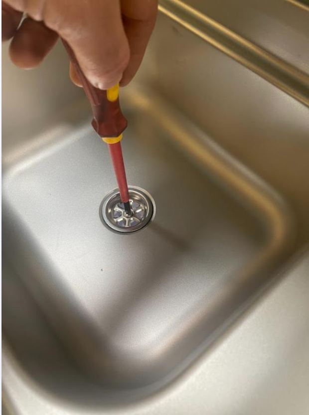
Screw the drain into place
