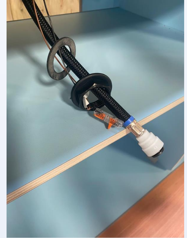
Feed the rubber seal then fixing thread over the water pipe and cables from behind and tighten
