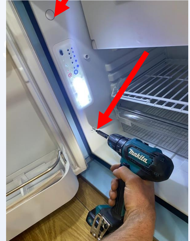
Remove the fridge fixing point caps, screw through into the aperture, use 30mm screws, be mindful not to screw through the ply
