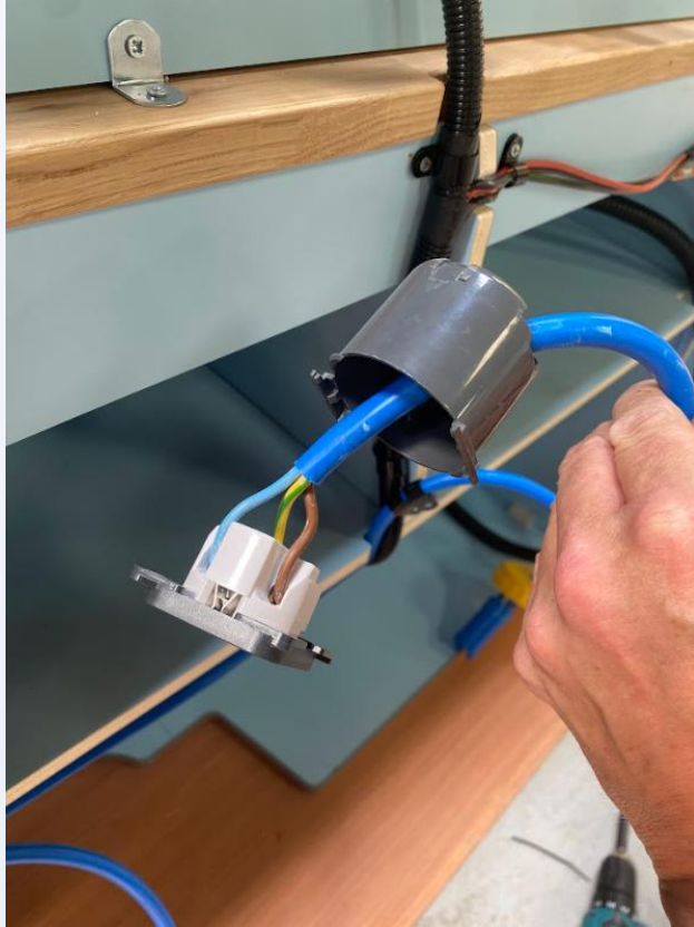
Remove the back cover of the 240 C-line socket
