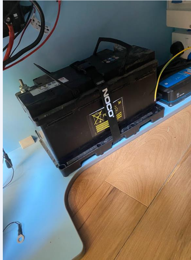
Fit the battery to the stary and secure with the strap
