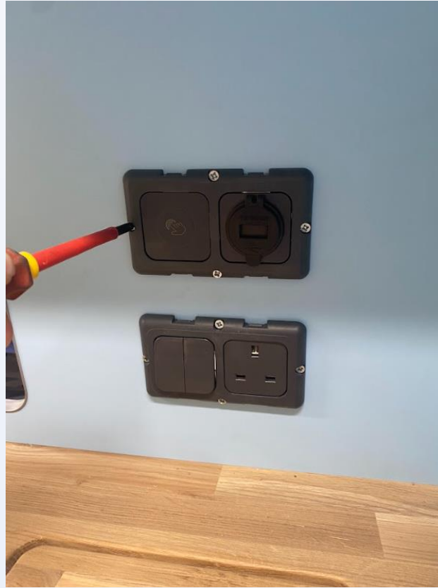
Clip the controls into the fixing plate then screw into place aligning with the pilot holes provided
