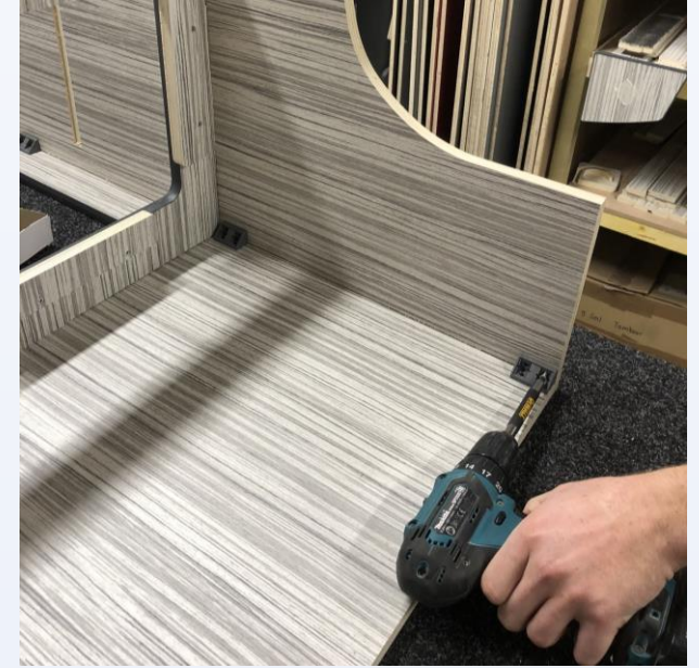
Fit the wardrobe upright (L) first, align all rebates and start from the base working up to the top using the blocks and pilot holes
