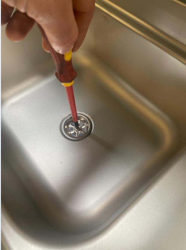
Screw the drain into place
