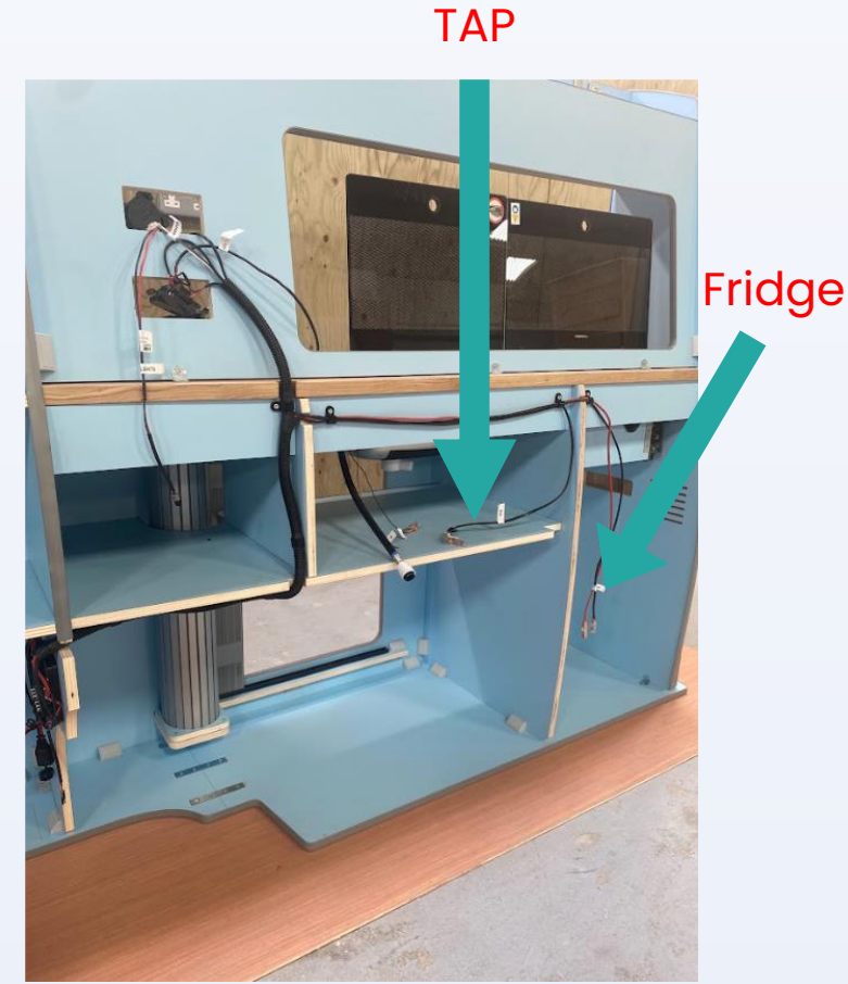
Using the cut outs in the furniture, run the fridge and tap cables into place and p clip into position
