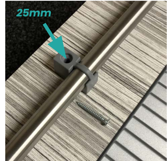
Fit the center support using a 25mm screw
